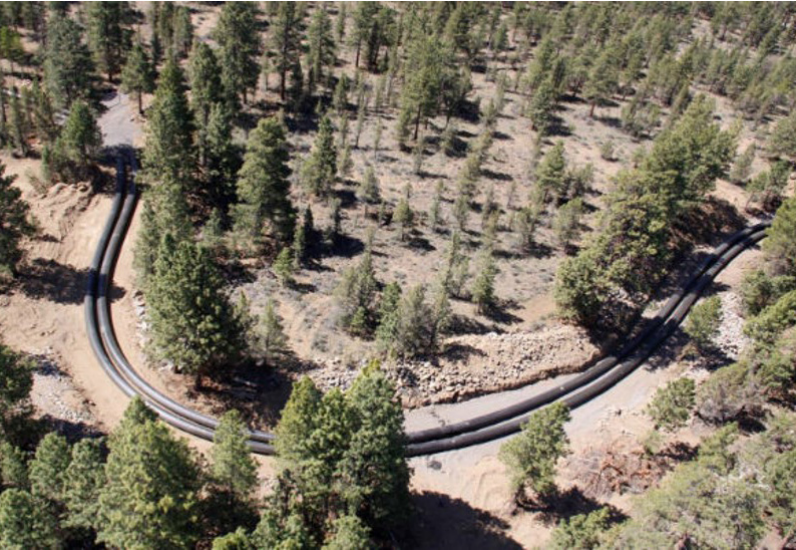
HDPE pipe installed at Oregon's Three Sisters Irrigation District.
